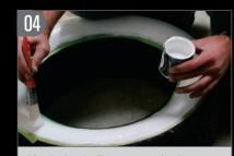
After letting the first coat cure for the recommended 24 hours, we applied a second and third coat in 24-hour increments as the manufacturer suggested.
