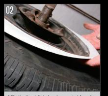
With the tire deflated and separated from the wheel, we fit the Port-A-Wall around the wheel and centered it accordingly.
