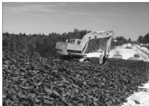
Use of tire shreds in civil engineering fill on Route 9, Days Hill, Maine. Source: Dana Humphrey.
