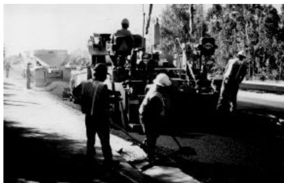
Application of rubberized asphalt concrete in Sacramento.
